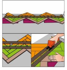
Leave the end-panels uninstalled. Tape along the marked line and place the flooring on top of a few flooring packages. Cut along the marked line with a jigsaw. Make sure that the click connections dont loose.
